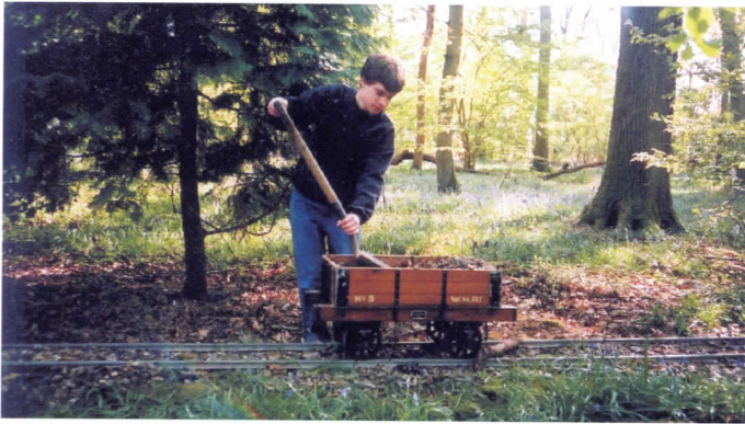
Philip Cracknell rebalasting the track in the woods.
