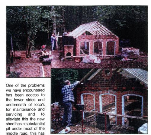
however been used as a swimming pool by the wildlife over the summer but is now dry thanks to an overall waterproof membrane beneath the floor slab and the side walls.
