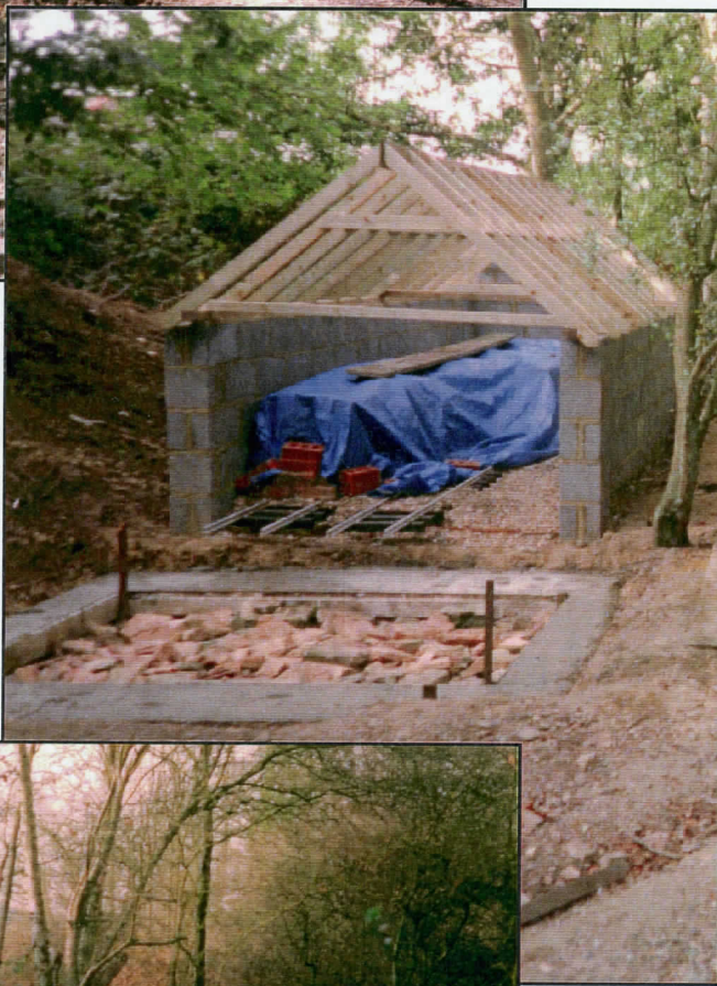
Right: The concrete carcass of the new carriage shed takes shape
