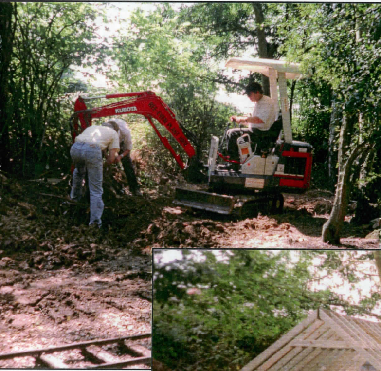
Above: The troublesome tree stumps are removed
